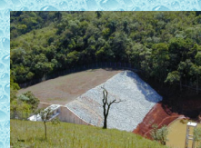
Dam: made of earth to form a reservoir as source of water
