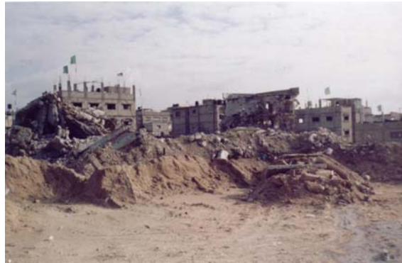
Figure 3. Demolished houses in Rafah
